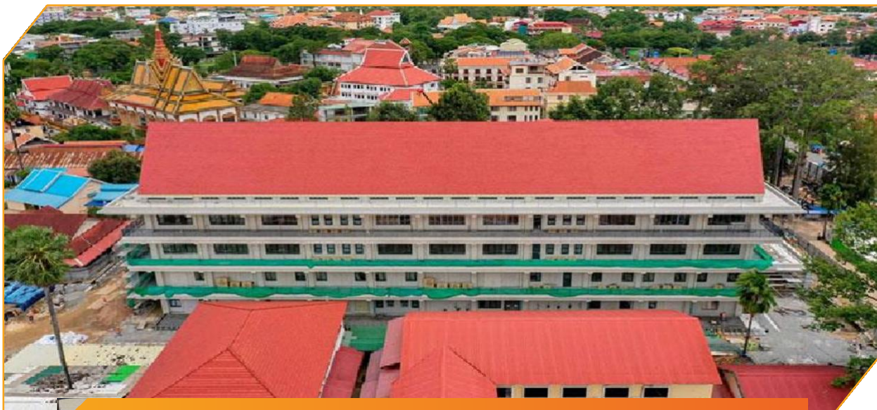
The Project for Improvement of Referral Hospitals
