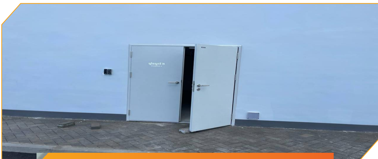
Steel door, shutter door work
