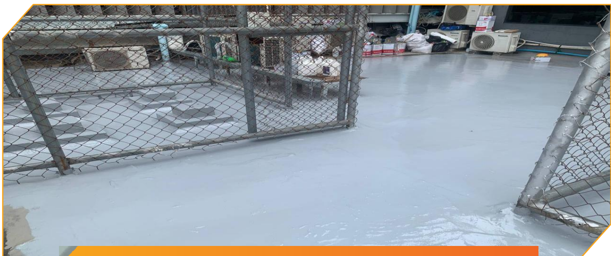
Waterproofing work for Head Office
