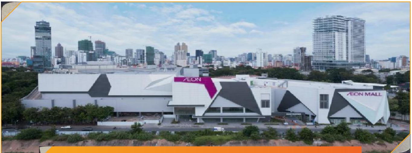
AEON MALL PhnomPenh Renewal and Extension
